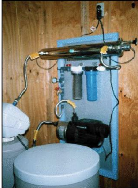
Figure 3.1 Example of UV treatment setup
